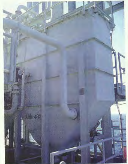
Fig. 1—A corrugated plate interceptor.
