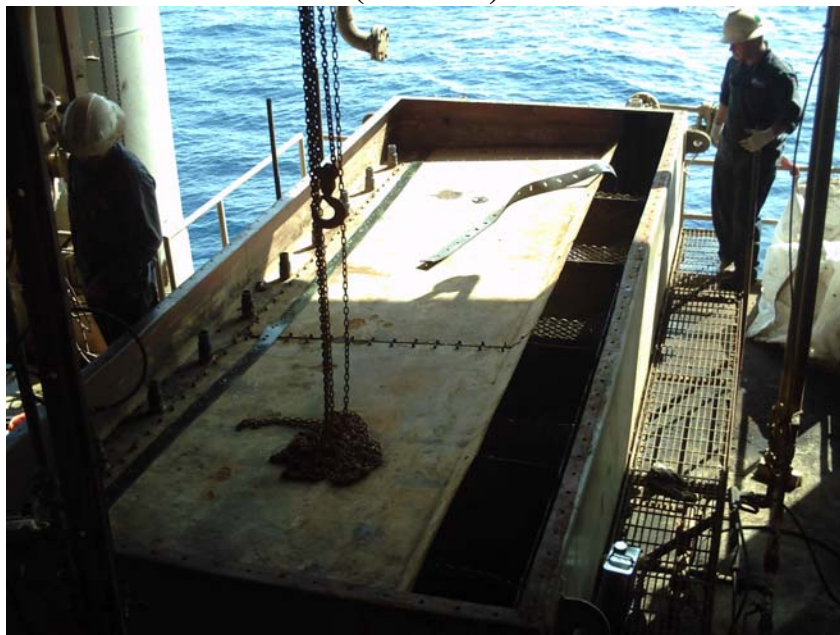
The picture shows installation of the baffle Plate and Eductors
