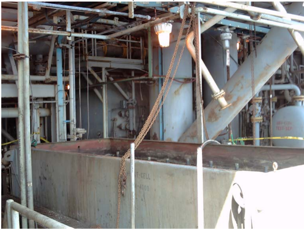
Starting to disassemble the existing IGF
